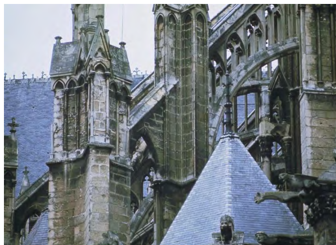
Figure 2.6 : Flying Buttress (Amiens Cathedral, 1862)
