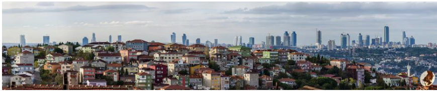
Fig. 1. Excessive construction activity in Istanbul.
