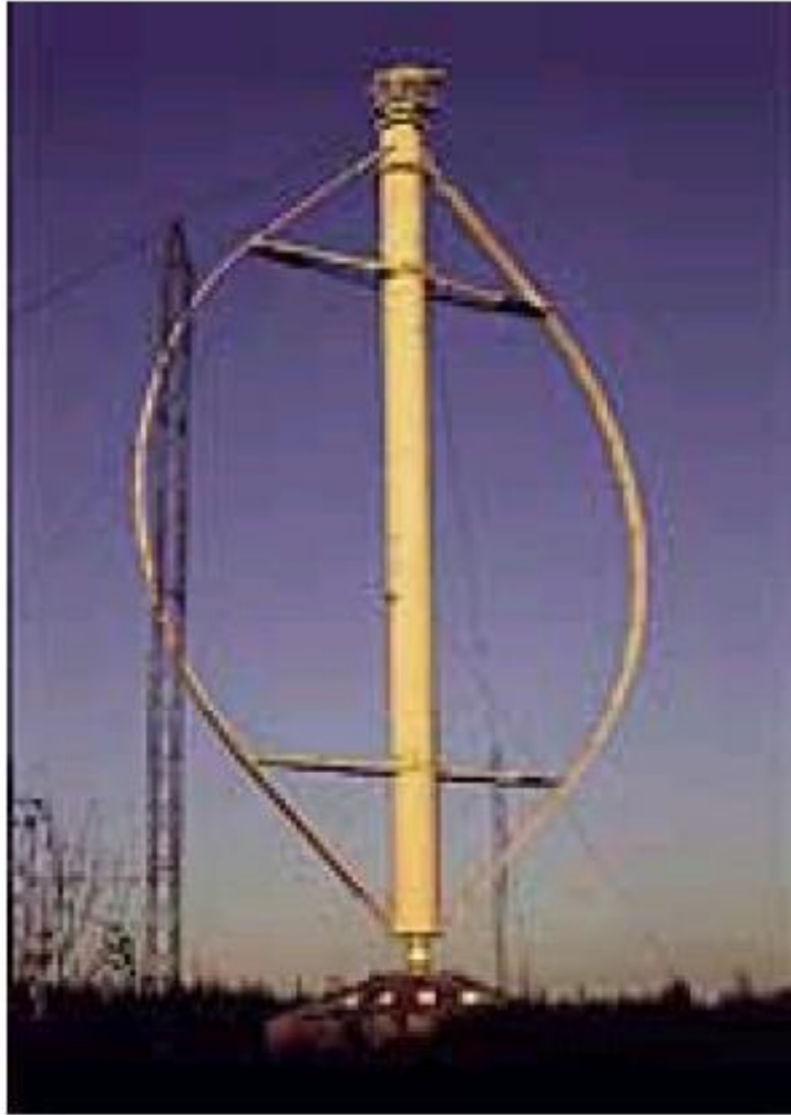
Figure 1.1 Eole C, a 4200 kW vertical axis Darrieus wind turbine with 100 m rotor diameter at Cap Chat, Quebec, Canada. The machine, which is the world's largest wind turbine, is no longer operational [3].
