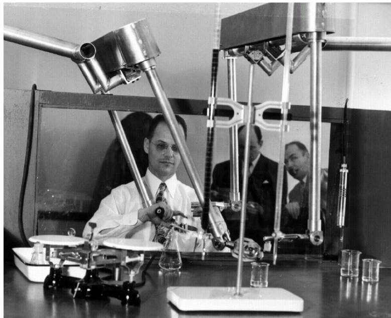
Figure 1-1 First mechanical master slave manipulator by Ray Goertz [11]
