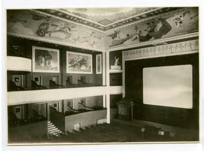
Figure 2.6 An inside view of the Süreyya Cinema House, originally and now an opera house in Kadıköy, Istanbul: Gökhan Akçura's Archive
