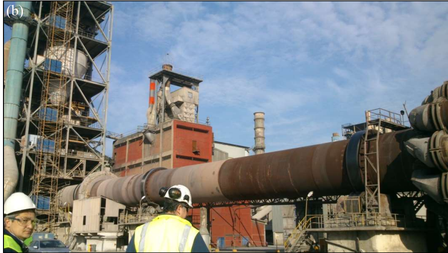
Figure 1.3. a) A schematic of rotary kiln with the pre-heater tower, clinker cooler and other sections [17], b) A rotary kiln in AkçanSA factory, Büyükçekmece, Istanbul.
