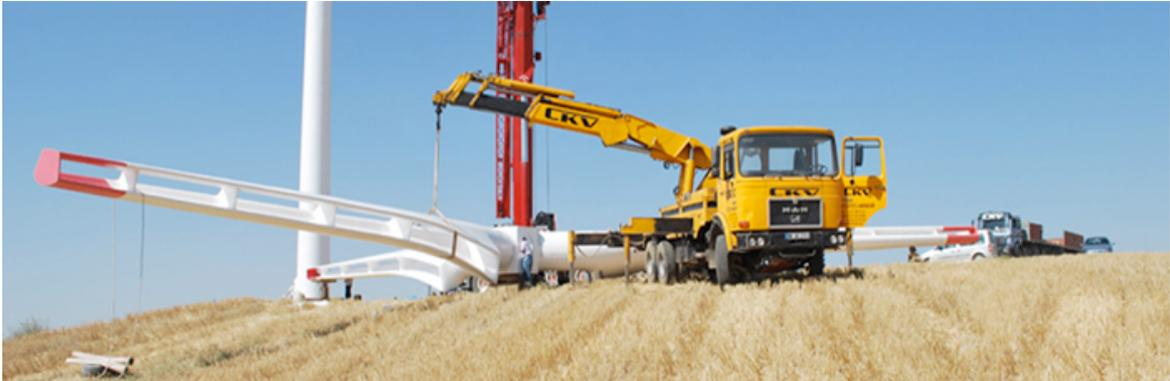
Figure 3 – Installation of the first 300 kW wind turbine developed in Turkey [9].
